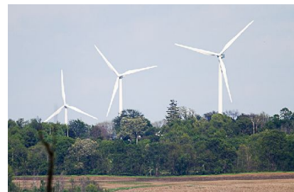
Wind Turbines near Horicon
